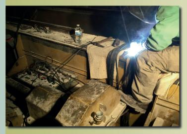
In another case one of our team was seconded on-site with the customer and worked with the team to complete a complex welding job. This involved removing magnetic fields of over 800 Gauss working several meters up on the crane gantry.
