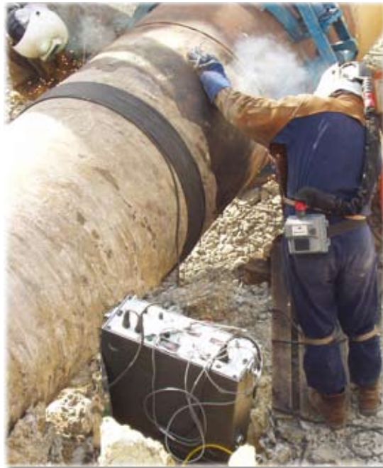
Fig. 2. Demagnetising a gas pipeline
