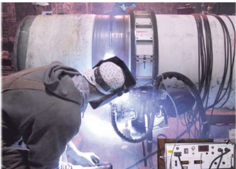
Fig. 1. Zeromag in use on an underground pipeline.
