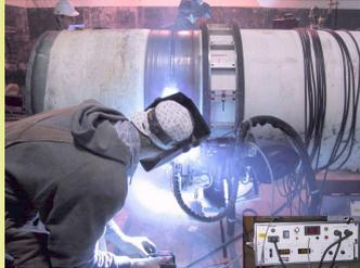
For any demagnetizing job, it is essential to understand the magnitude and sign of the magnetic field; this then allows an informed choice of demagnetizing method. The Diverse Magmeter MF300H+ is a robust tool for measuring magnetic fields at the ends of pipes or in narrow weld preps. Rather than using a delicate ceramic detector, the MF300H+ uses a high performance semiconductor encased in stainless steel.
