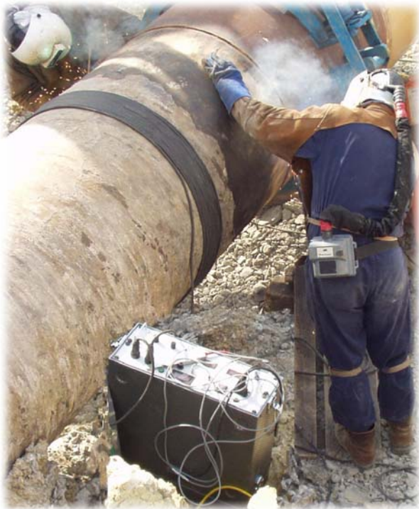
Fig. 2. Demagnetizing a gas pipeline
